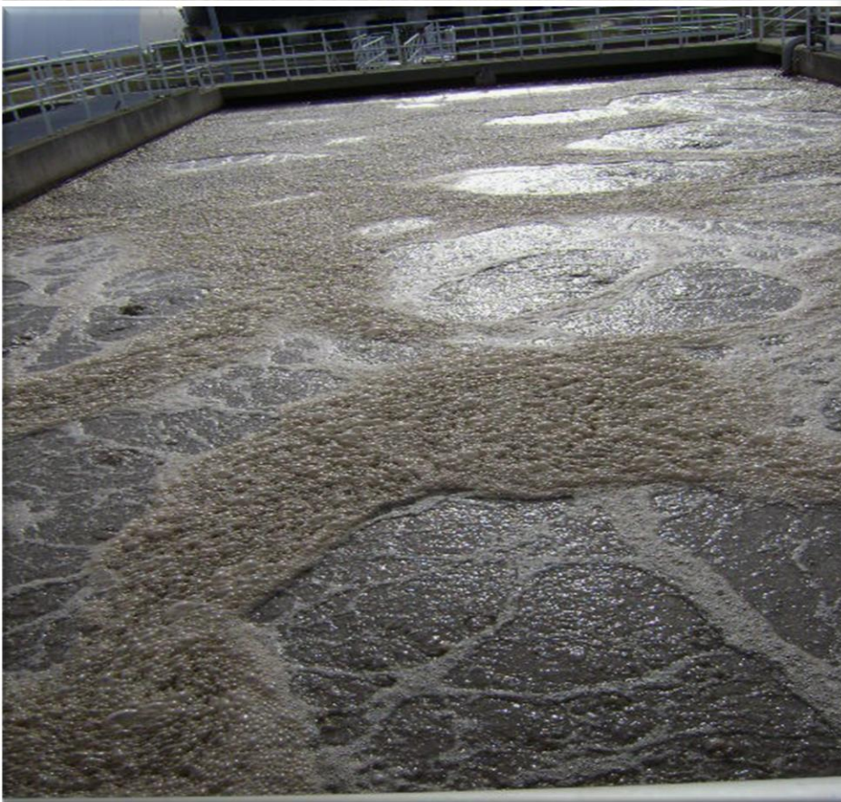
Foaming on Aeration Tank
