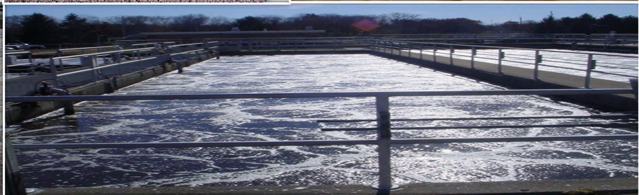
Foaming on Aeration Tank
